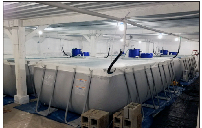
Figure 4. Swimming pools being used as shrimp tanks in an indoor, insulated facility. The blue drums are filters, netting prevents shrimp from jumping out of the tanks, and blown air is delivered to diffusers through the PVC piping.
